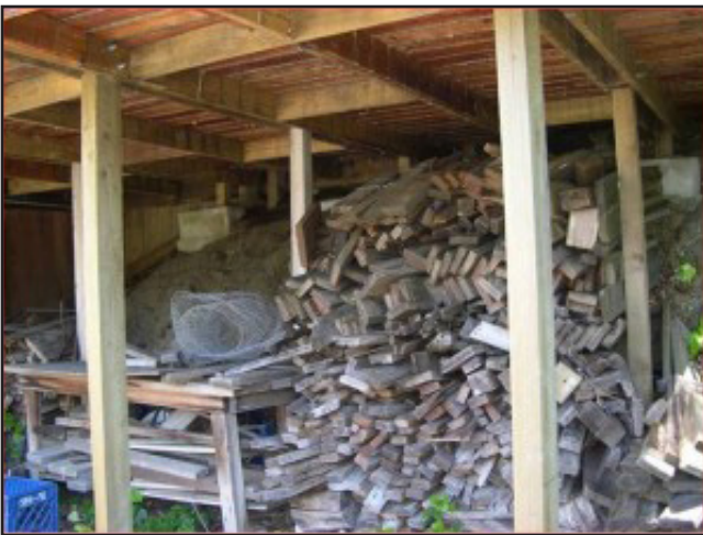
No deck, regardless of the material used to build it, would be safe if this amount of fuel beneath the deck caught fire. Even decks that may have a noncombustible surface, such as concrete, use lumber and timbers for structural support and those materials can catch fire.
