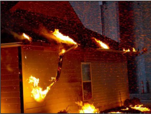
This photo shows how gutters filled with debris can be ignited by wind-blown embers that land there. Once ignited, the edge of the roof and fascia are exposed to direct flame contact.
